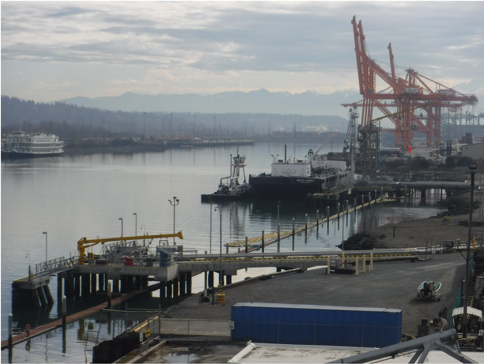
Figure 5: Looking Plant South from Dock 2 to Dock 1
